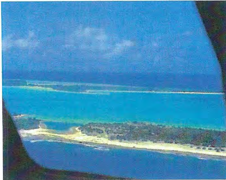
FIG. 17.21. The never-completed submarine channel started at the beginning of WWII, through the middle of Wilkes Island. Peale Island in background across the lagoon
