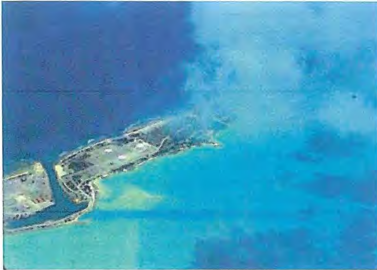
FIG. 17.22. The small boat harbor was originally open to the lagoon but was sealed by construction of a seawall. The small boat channel that was once used is evident but was closed off when the causeway connecting Wake Island (left) to Wilkes Island (right, with the three fuel storage tanks) was constructed. The overall best diving was in the immediate area on the outside reefs by this harbor. The wreck of an oil tanker is in shallow water by the harbor entrance and is colonized by corals
